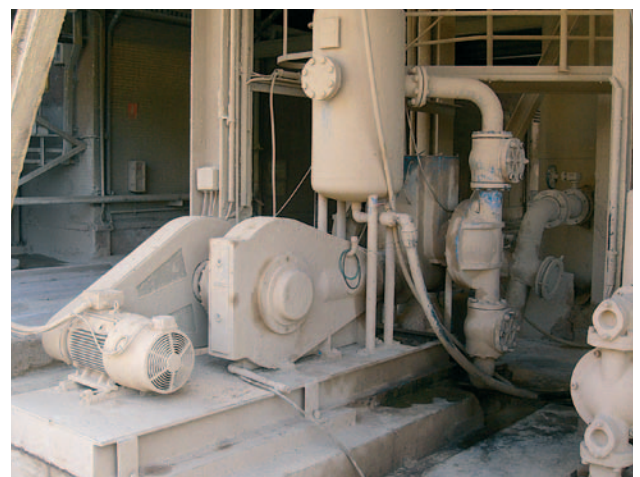
ABEL HM for transfer of ferrous jarosite sludge
