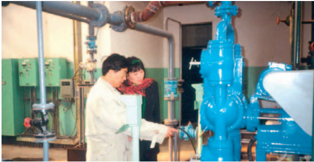
ABEL CM-pump for spray dryer feed
