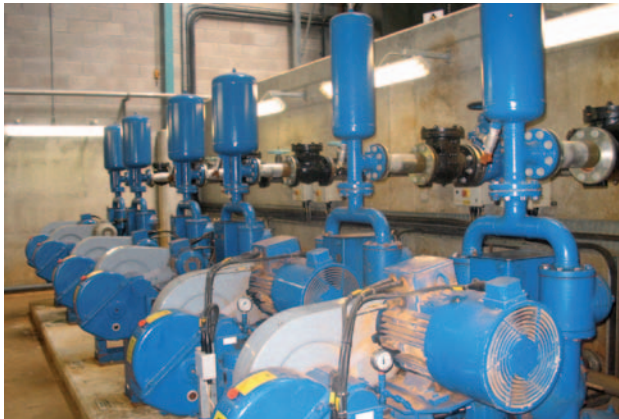
CM piston diaphragm pumps in a water treatment works in Northern Ireland
